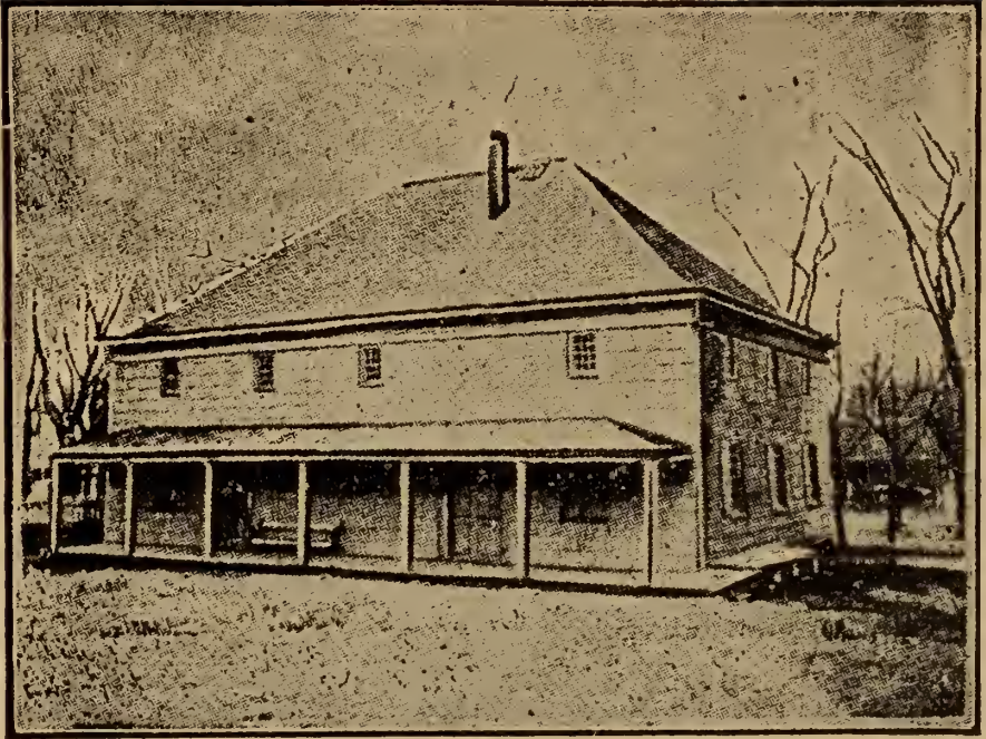
FRIENDS MEETING HOUSE, FLUSHING. BUILT 1695.
